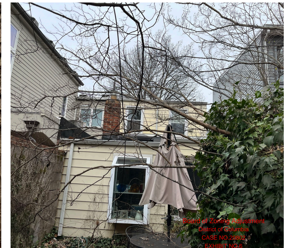
EXISTING REAR FACADE
