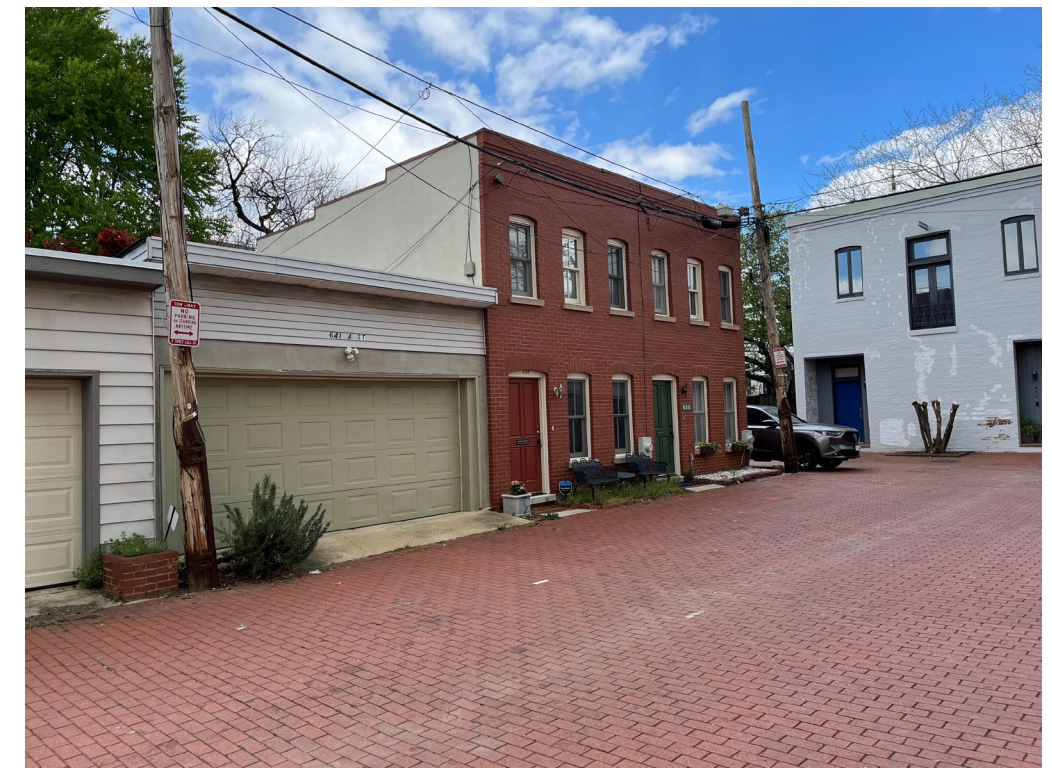
REAR VIEW LOOKING EAST
