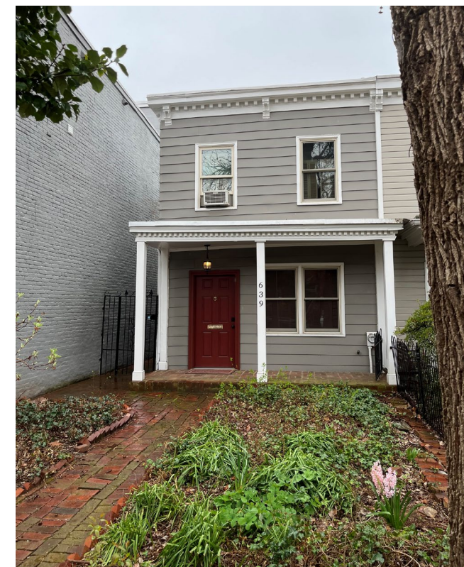
EXISTING FRONT FACADE
